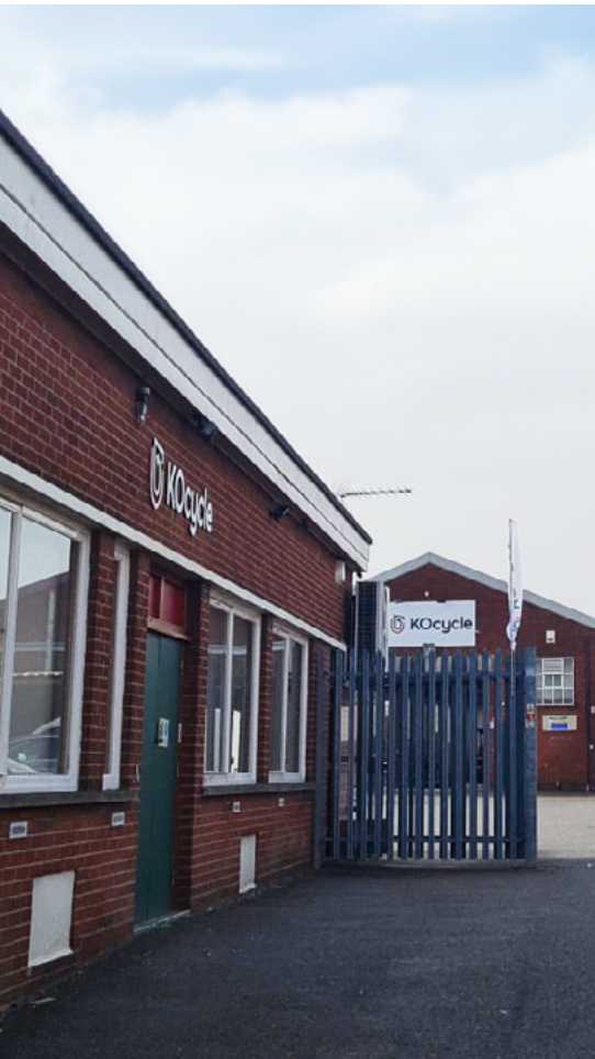
KOcycle's new hardened operations facility in Braintree features over 30,000 square ft of operations focused on security and sustainability.
