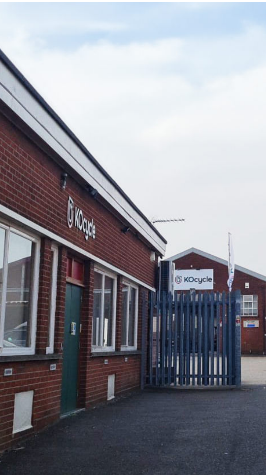
KOcycle's new hardened operations facility in Braintree features over 30,000 square ft of operations focused on security and sustainability.
